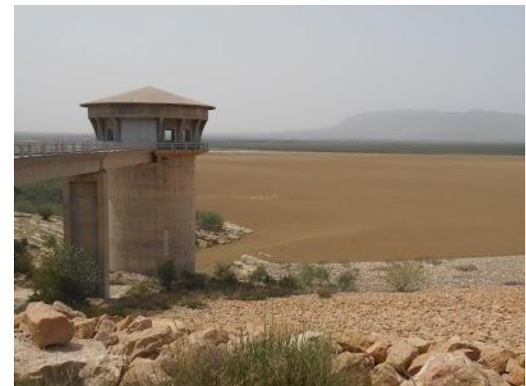
Dam El Houareb, 13/07/2017
