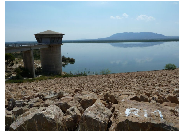
Dam El Houareb, 31/05/2012
