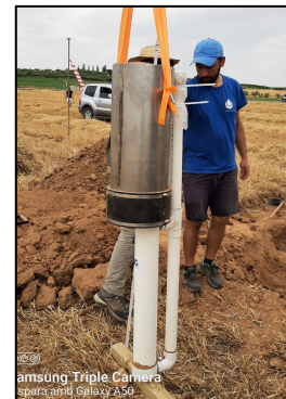
G3 lysimeter being installed
