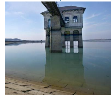
Ebre dam, Spain, 2017
